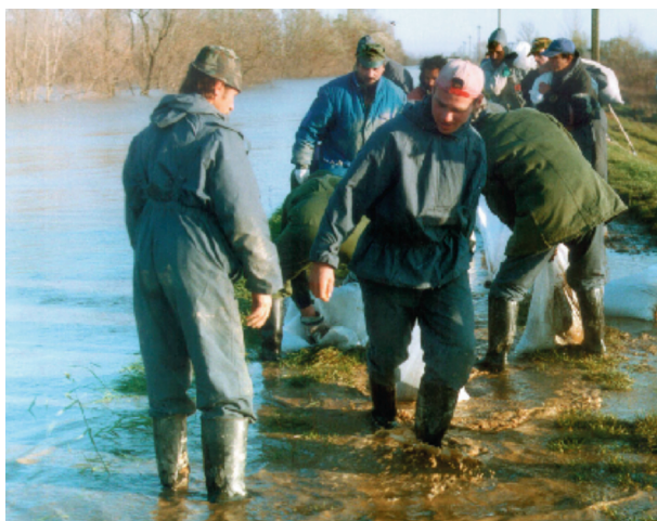
Increasing the height of the dike at overtopping water
