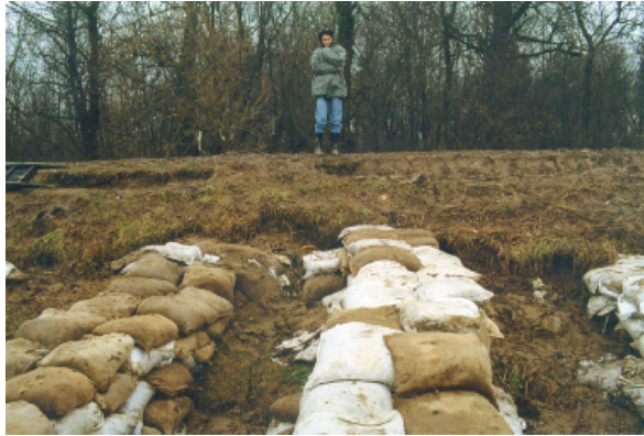
Construction of an excess weight band at the slough at Tarpa along the frontier at night on 7th November 1998.
