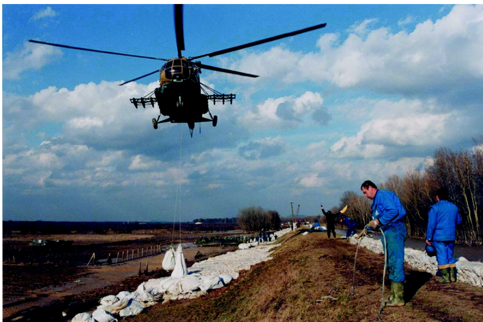
Helicopters assisted at the construction of the excess weight stone band
