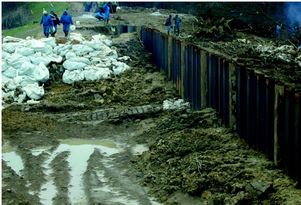
Completed blockage by sheet piling at 12+400 left bank section of the Tur
