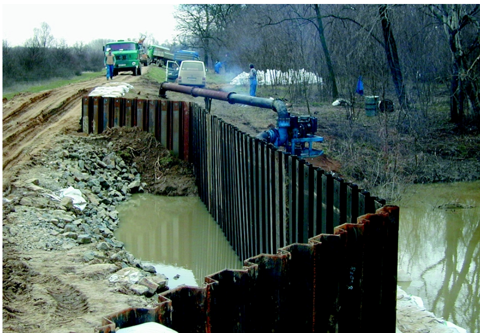
Completed blockage by sheet piling at 12+000 left bank section of the Tur
