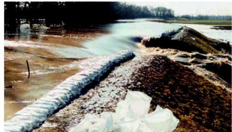
Process of the dike breach
