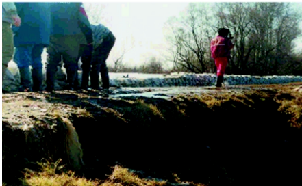
Process of the dike breach
