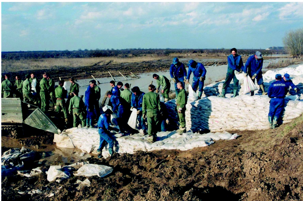
Constructing excess weight stone band with the help of the army
