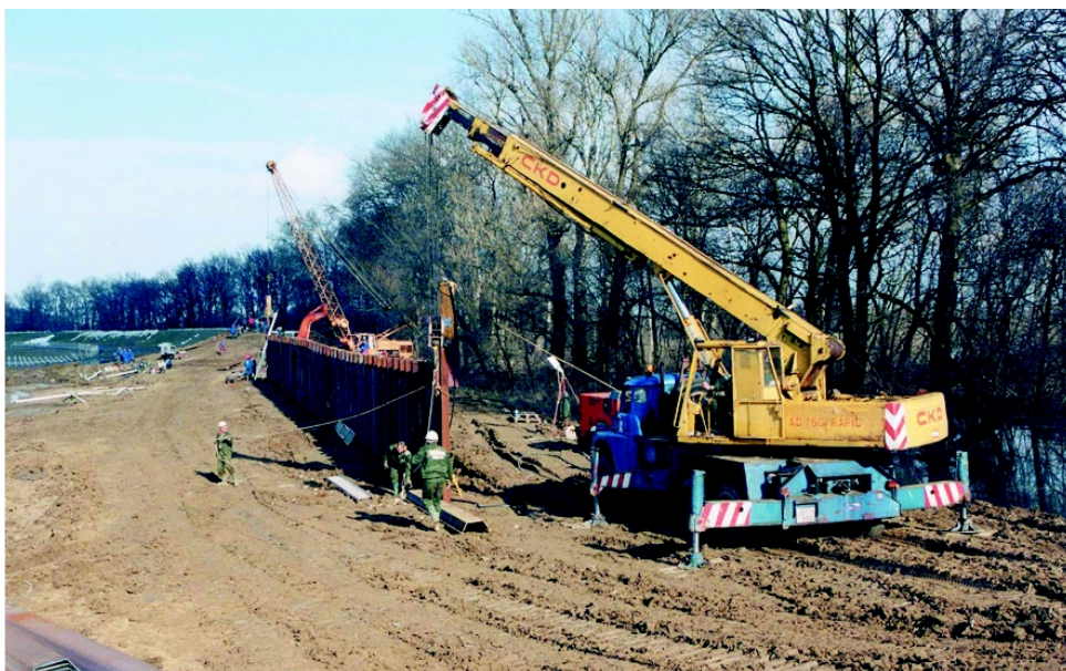
Sheet piling of the downstream dike breach
